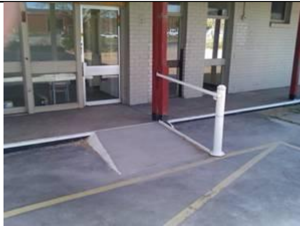
The new Access Ramp ready for business!
