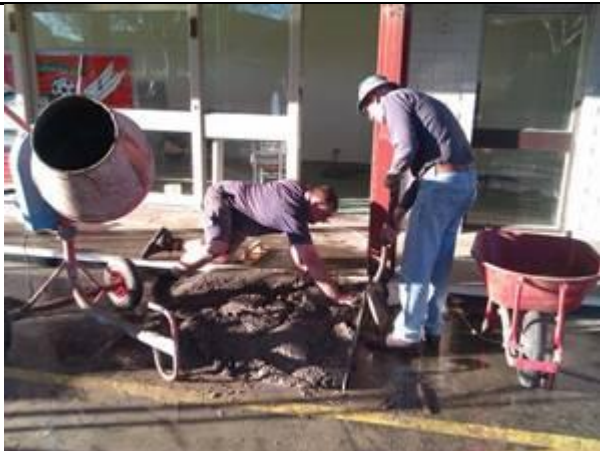
Al Phemister and Roger Holgate pouring the wheelchair access ramp
